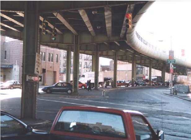
Figure 1 View of original bridge looking east along Borinquen Place
