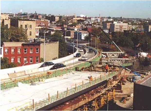
Figure 4 View of precast superstructure near completion
